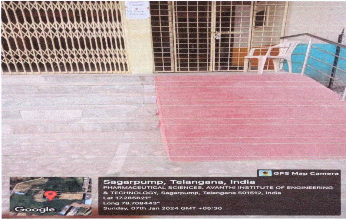
Ramps for Disabled Friendly Environment
